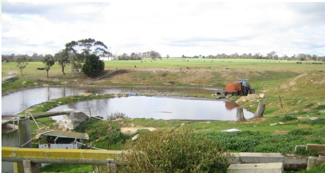
Wastewater Dam System including Anaerobic and Facultative Dams
