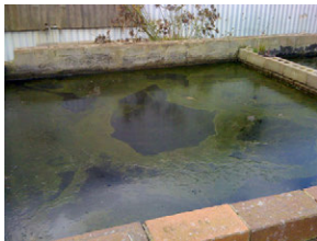
1,300Gal (5,000L) fresh water tank, prior to the application of BiOWiSH™, showing inlet (far left, with float / ball valve) and linked sections, all with moderate to severe algal growth on the surface of the water.
