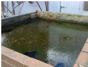
1,300Gal (5,000L) fresh water tank, prior to the application of BiOWiSH™, showing inlet (far left, with float / ball valve) and linked sections, all with moderate to severe algal growth on the surface of the water.
