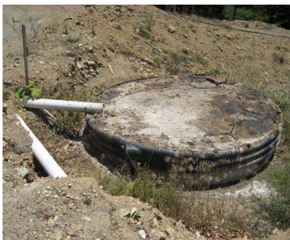
Tallow Dam Before Severe crusting on the dam is causing effluent to run off onto the ground surrounding the dam, rendering it useless.
